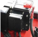
All the controllers, relays, and safety fuses are allocated in the controller box, free to water and dust.
